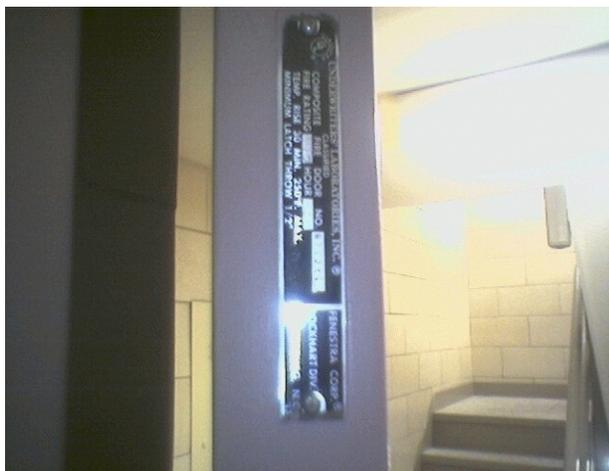
To the left is the testing laboratory's label on the inside edge of the door indicating that it is properly rated as a fire door. Fire doors must be certified by recognized testing laboratories (such as UL) and must have the laboratory's certification label on the edge.
